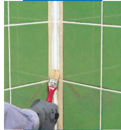
Smoothing the joint with soapy water and a small brush
