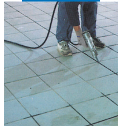
Sealing ceramic tile floor with Mapesil AC
