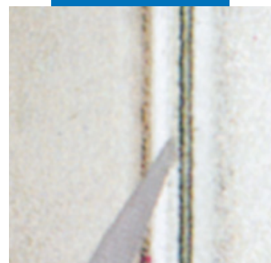
Sealing U-profile glass
