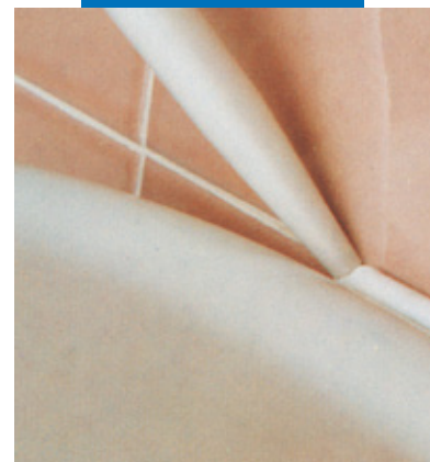
Sealing sanitary ware
