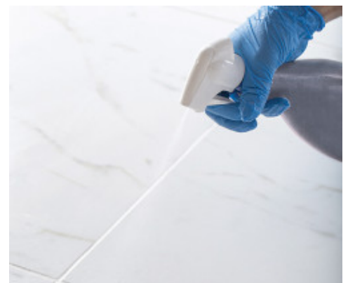
Possible final cleaning with UltraCare Kerapoxy Cleaner
