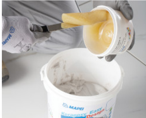
Pour the hardener (component B) in the container of component A
